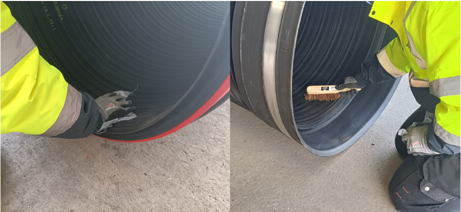
Figure 4 Cleaning pipe end with rag (left) and brush (right)
