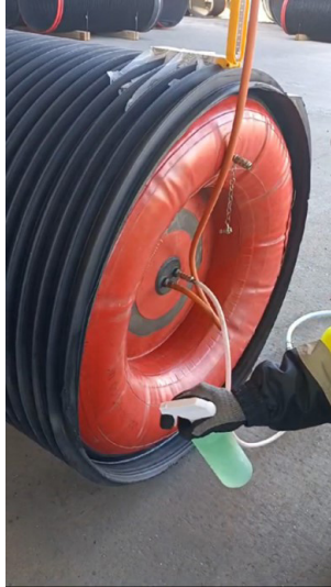
Figure 10 Picture of soapy water being applied to the inflatable bung to check for air leaks
