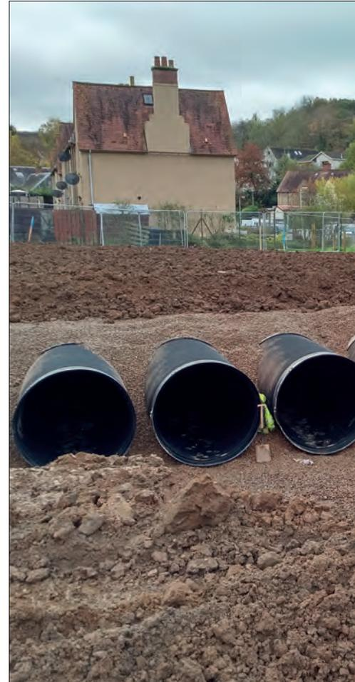
port manifold. The inlet pipe connects into the upstream end of the first pipe only, which effectively converts the first pipe into the primary, combined carrier and storage pipe, with the remaining six pipes functioning as secondary storage pipes at times of peak discharge.
